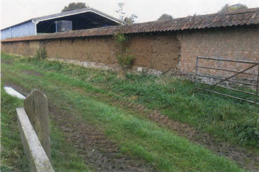
Fig. 7 Tile-capped wall with 'mud-walling' stretches, Home Farm, Rearsby
