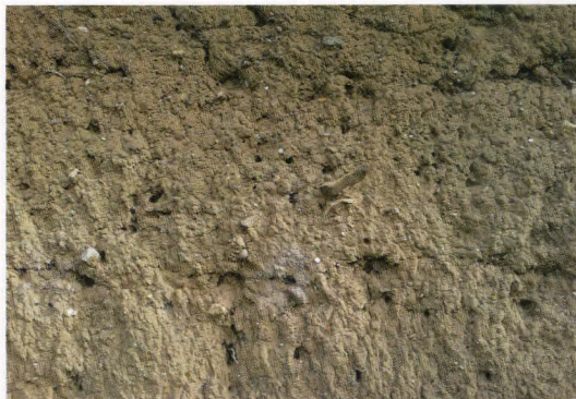
Fig. 8 Detail of 'mud-walling', Home Farm, Rearsby
